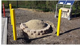
Figure 3. Subsidence at EOCG. Note the seismic vault has clearly subsided, and the yellow posts have been recently installed. Photo courtesy of Dan Determan, USGS. Photo taken on January 6, 2015.
